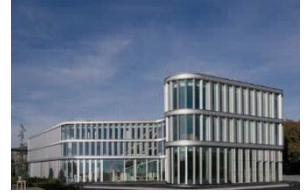
The NanoFactory building in Haar – a hotbed of technology on the east side of Munich.
